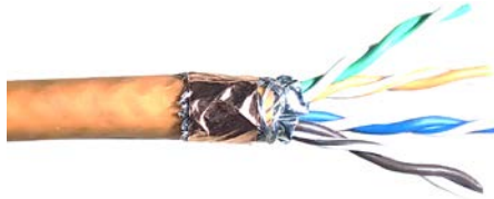
④.4.Fan out all four twisted pairs, allocate each by following colorcoding label
